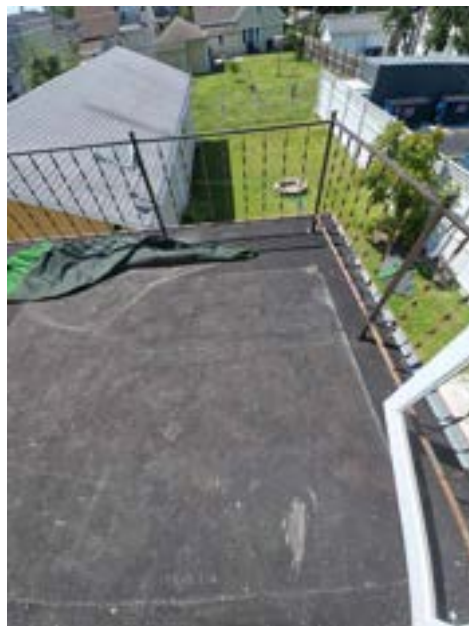
Rubber roof at balcony porch
