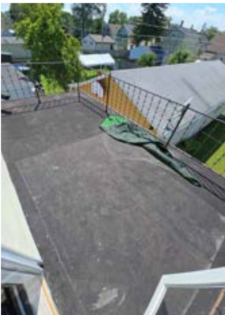
Rubber roof at balcony porch
