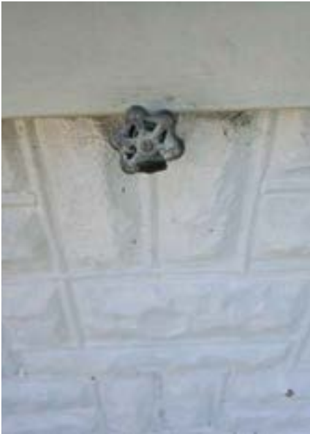
Damaged handle
