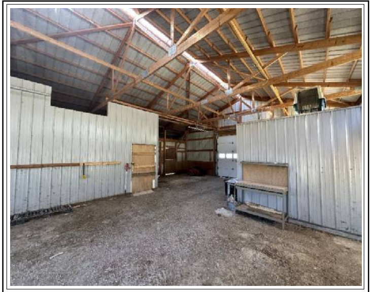
INTERIOR OF SHED
