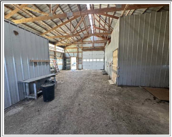
INTERIOR OF SHED
